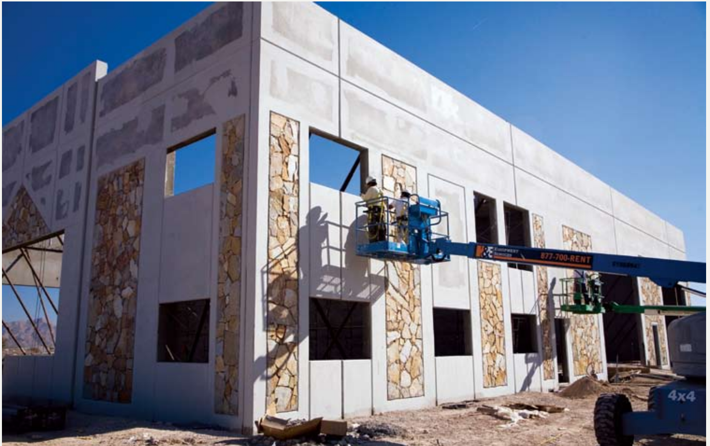
At American Stone's two-story showroom, LM Construction is using tilt-up walls with poured in place stone panels.
